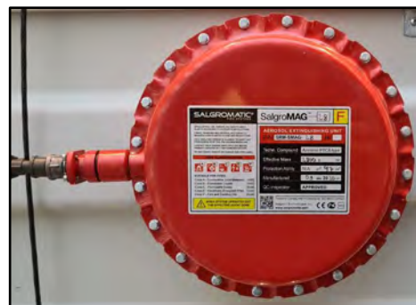
Figure 2: EP203 control panel, fire detection and Salgrom SRM-MAG.
